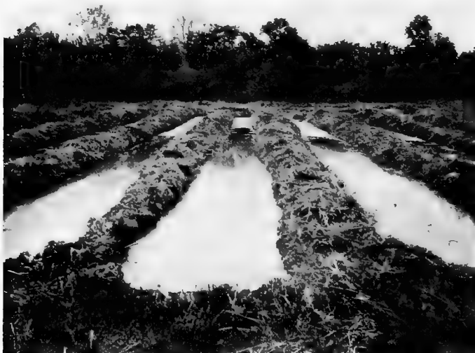
Fig. 42.—Surface disposal of sewage—a crude system.
